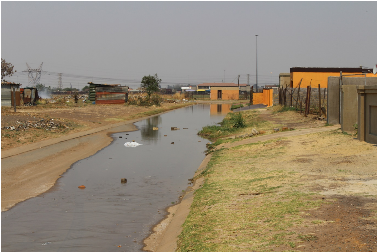
Above: Sewage running through Mongau Street, Tshepiso, Sharpeville.
