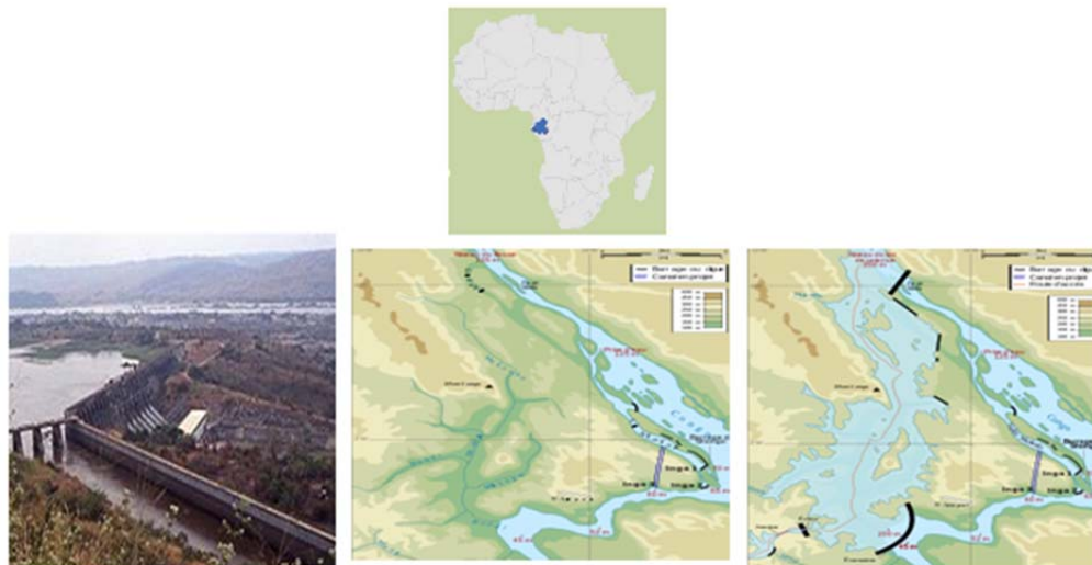
Figure 40. Inga I dam, with the feeding canal for Inga II in the foreground
