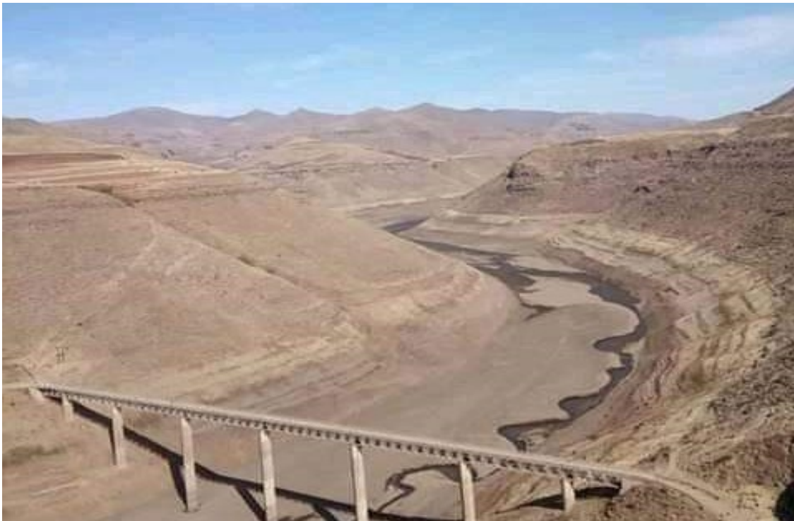
Figure 9: An alarming sight – a very dry Katse Dam in September 2019 – level at 16.9%
