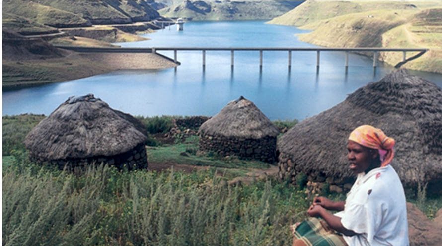
Figure 2: Katse Reservoir with Katse to Ash River tunnel intake tower in background (Photo Aurecon)
