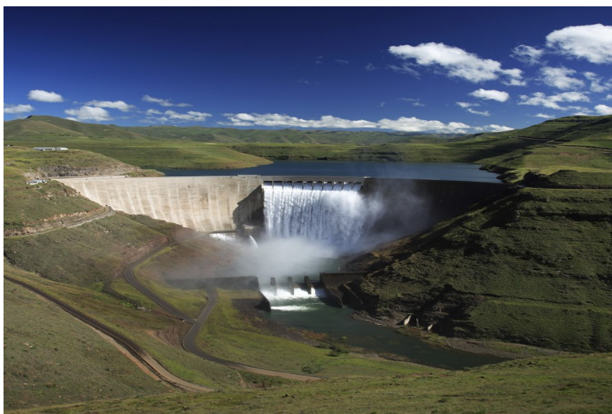
Figure 3: LHWP Phase IA Katse Dam wall (Photo Aurecon)
