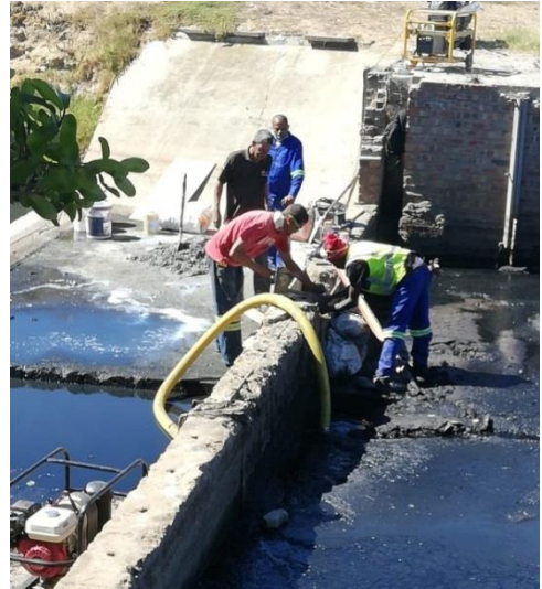
Weir repairs on 1 April 2020
