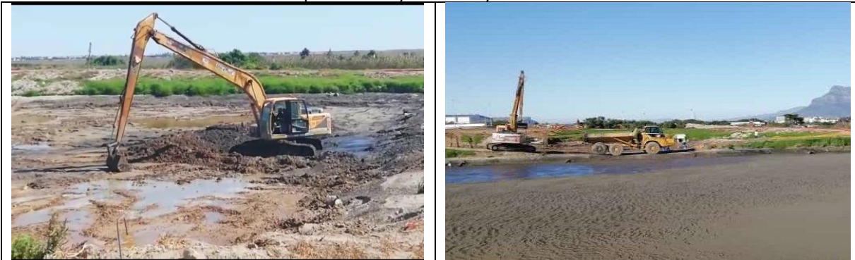
Cleaning of sludge from Dam 3, Potsdam Wastewater Treatment Works
