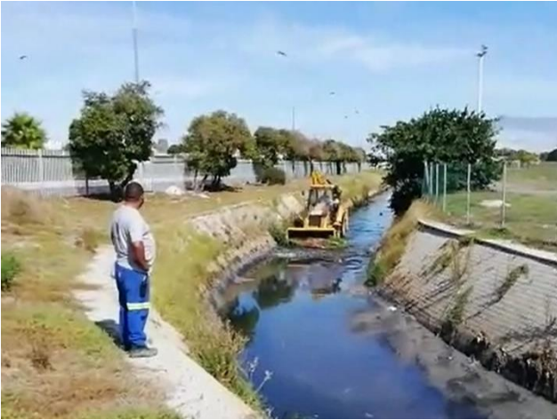
Sediment removal 19 April 2020
