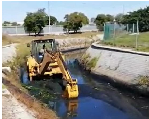
Sediment removal 19 April 2020
