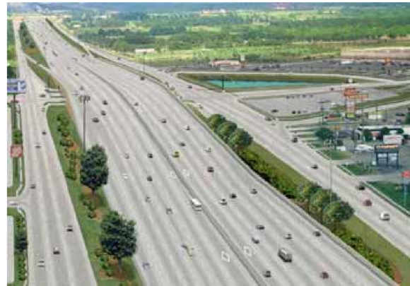
Katy Freeway at Fry Road after
