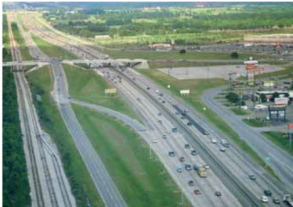
Katy Freeway at Fry Road before
