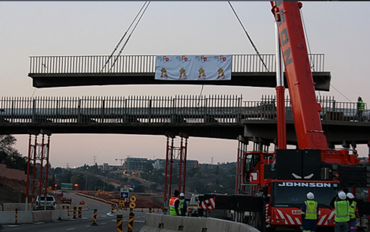
Demolish Bridge at Aitterbury Road: 14-15 Aug 09
