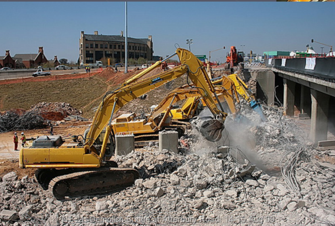
N1-21: Demolish Bridge at Atterbury Road: 14-15 Aug 09
